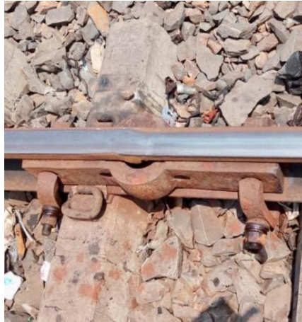
Figure 1: Rail Flaw Protected with Clamped Joggle Fish Plate
