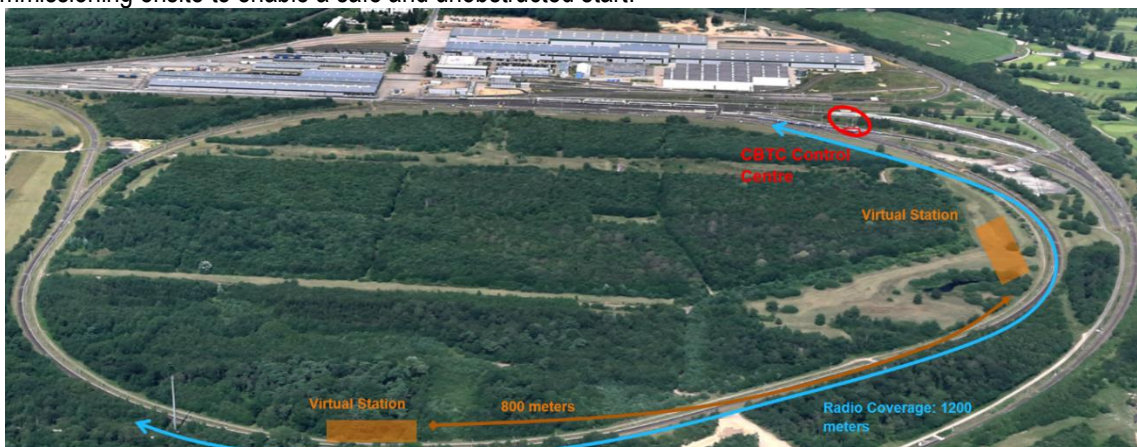
Figure 5: Riyadh Signalling Implemented on the Wildenrath Test Track – A purpose-built installation to enhance testing and reduce the amount access to the operational track
