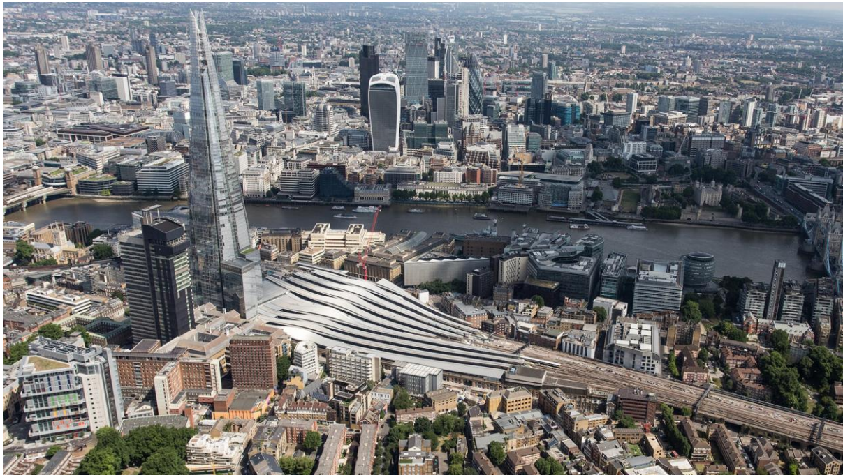
Figure 3: London Bridge – Showing the multiple track configuration – requiring stringent test and implementation
