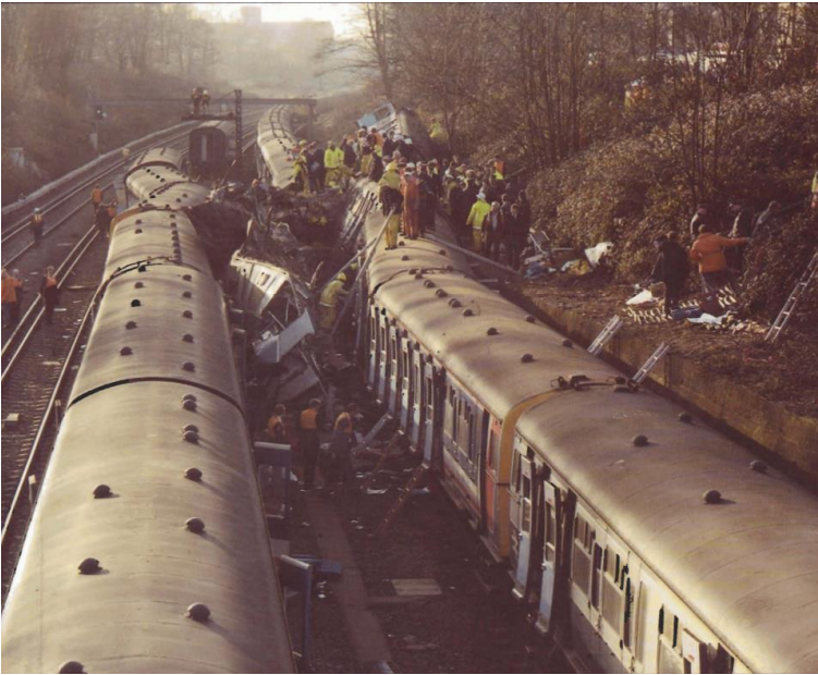
Source: Investigation into the Clapham Junction Railway Accident, Department of Transport (UK)
