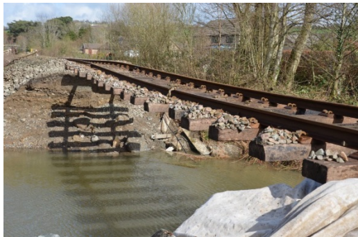
Figure 6: Conwy Valley line, March 2019
